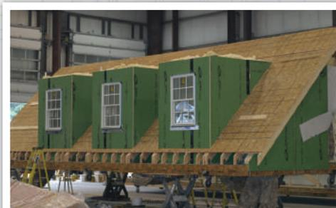
If you’ve ever shingled a roof or even watched it being done, seeing these professionals do it just makes you shake your head in wonder. They begin on a mezzanine level at exactly the level of the overhangs so they don’t have to step up too high to get on the roof. The mezzanine is fed with shingles from a forklift below. Also, the roof area is nearly flat now, since it is hinged in its lowered position (it will be tilted up to its
